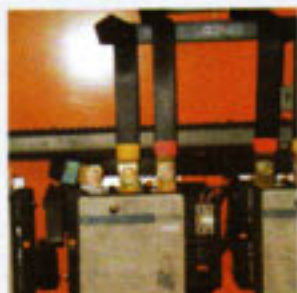
Electrical: Termination problem on yellow phase
